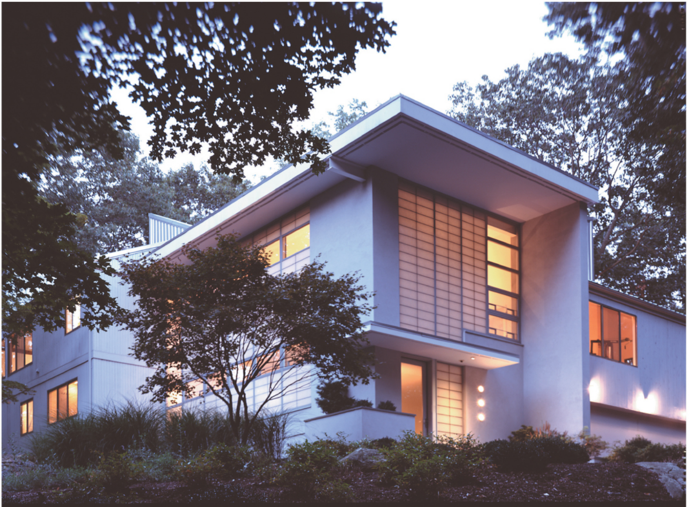
Top: Park Avenue loft, New York City. Photograph by Ake Eson Lindman Bottom: Pound Ridge House, Pound Ridge, NY. Photograph by Harry Zernike Opposite: Sagaponac House, Long Island, NY. Photograph by Paul Warchol
